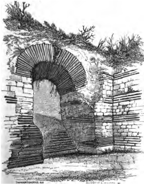
2. Forchester Castle, Hampshire. Roman Masonry and Arch formed of Roman bricks or tiles.
